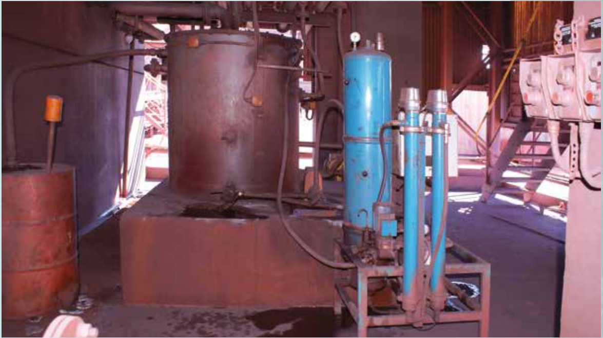
A CJC™ Filter Separator installed on one of the crushers at Kumba Iron Ore's Sishen Mine in the Northern Cape, South Africa
